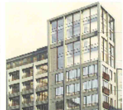
The added lower looks like a huge office (65)
